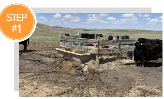
PREP: Clean out mudhole of mud, water, and slop. Scrape down berm and fill in mud hole, packing as you go. We use a skid steer to pack, driving back and forth with a scoop of dirt (for added weight), careful not to hit the tank.
