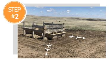
DRAINAGE: Create drainage spot, preferably on the low side of tank. We use a skid steer to dig a shallow ditch. This is to allow the majority of rain water or, if the float breaks, overflowing water to drain away from the
