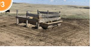
PACK: Pack dirt level with the bottom of the tank. Spread a layer of loose dirt or gravel on top of the packed dirt, approximately 2 inches is sufficient. Leave this dirt unpacked.
